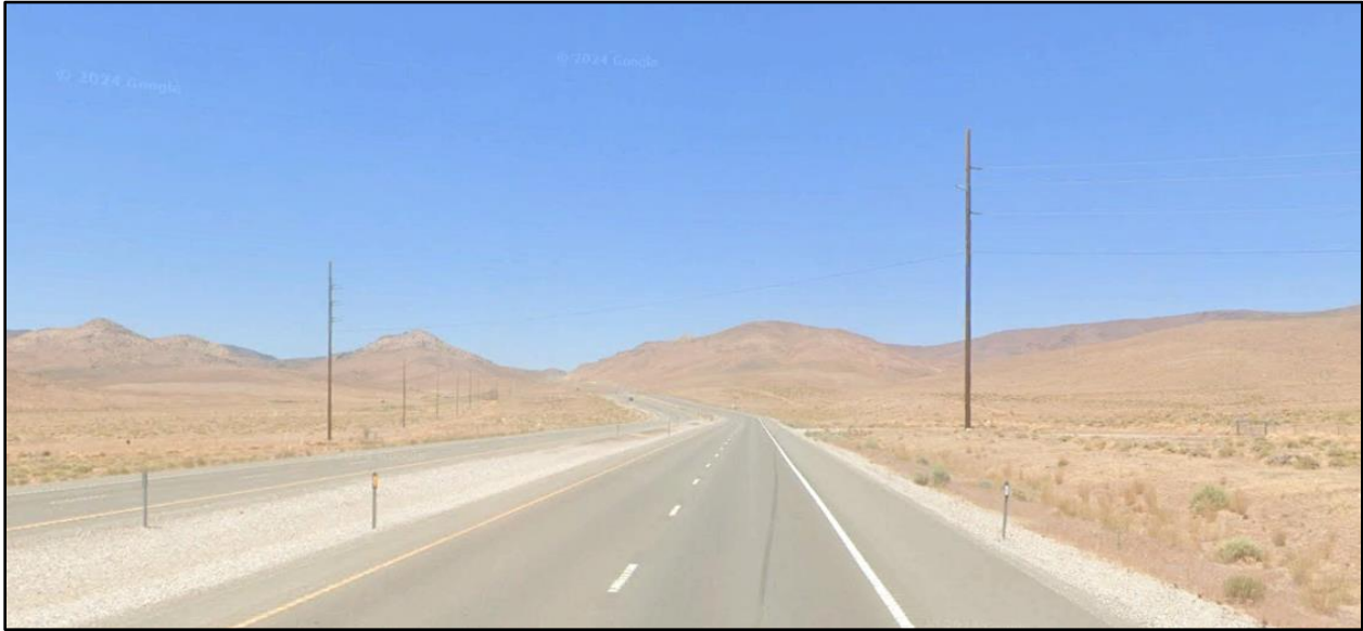
GoogleEarth Streetview Location 4 along USA Parkway – View Northwest
