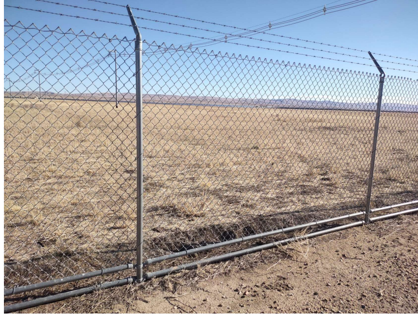
Topaz Solar Farm array fence, photo by Misha Allen
