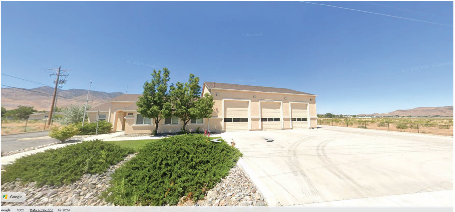
Figure 3 – Fire Station Street View
