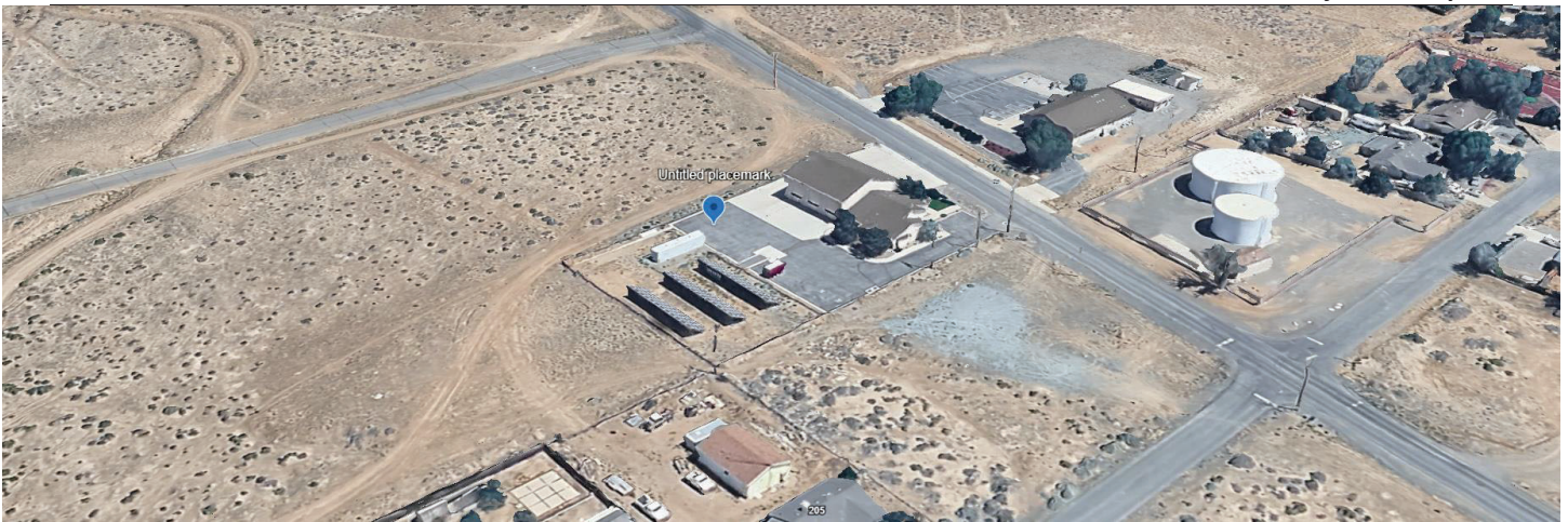
Figure 5– Fire Station Aerial View looking south-east toward US Hwy 50. Heli-base would be located on the blue pin on the north-east part of the fire station property.
