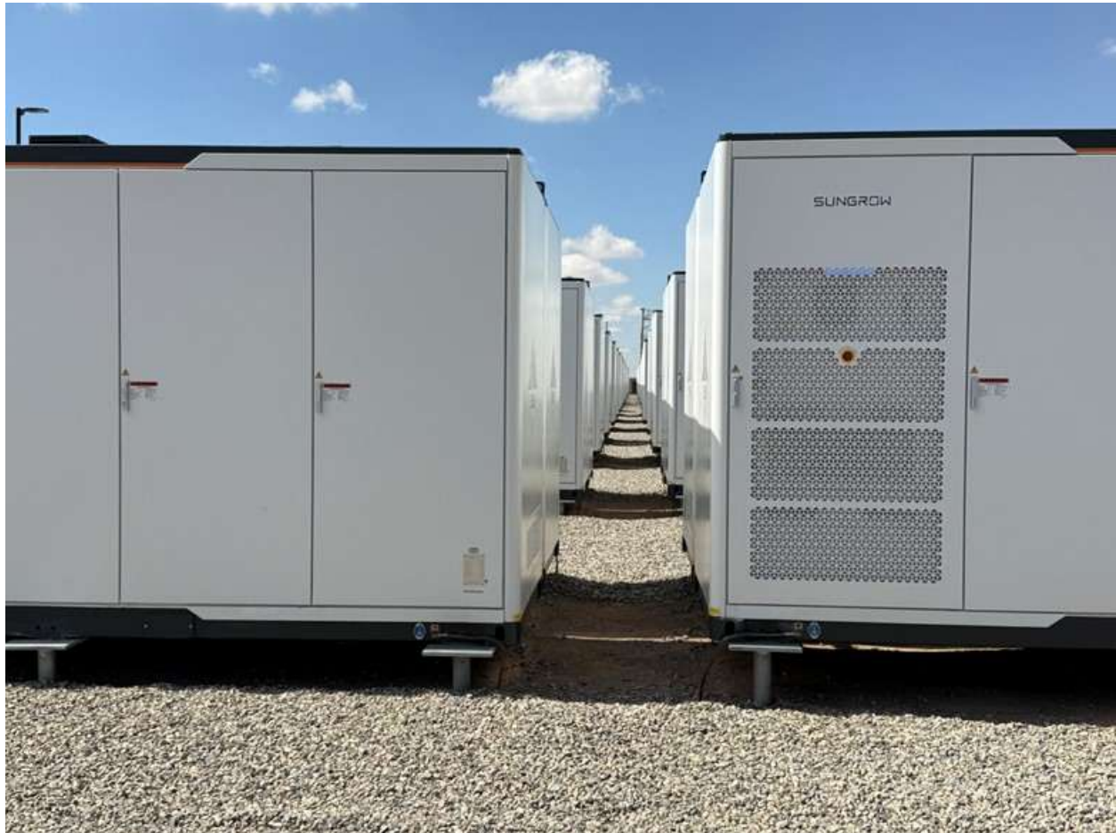
FIGURE 9: BATTERY ENERGY STORAGE SYSTEM ENCLOSURE
